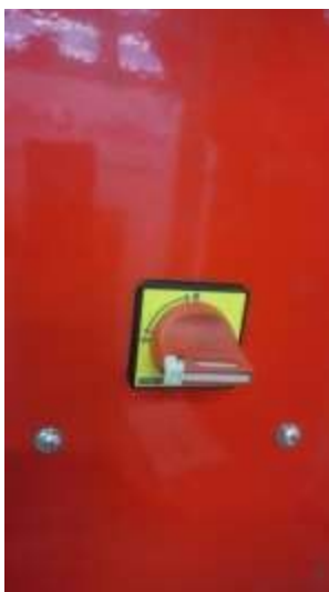
Pic. 7 Main power switch
